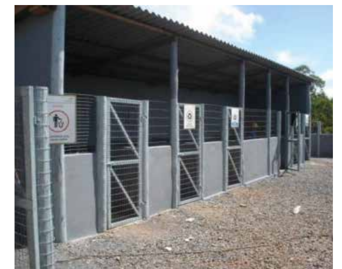
Central de Resíduos – UPE Burity
